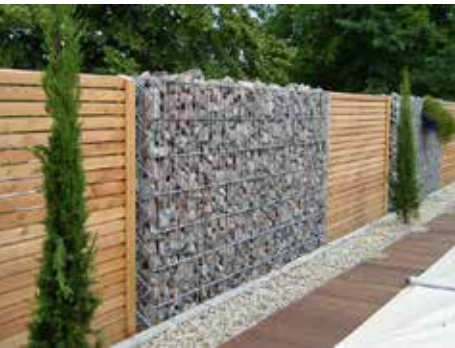
Gabion & Wooden Fence
