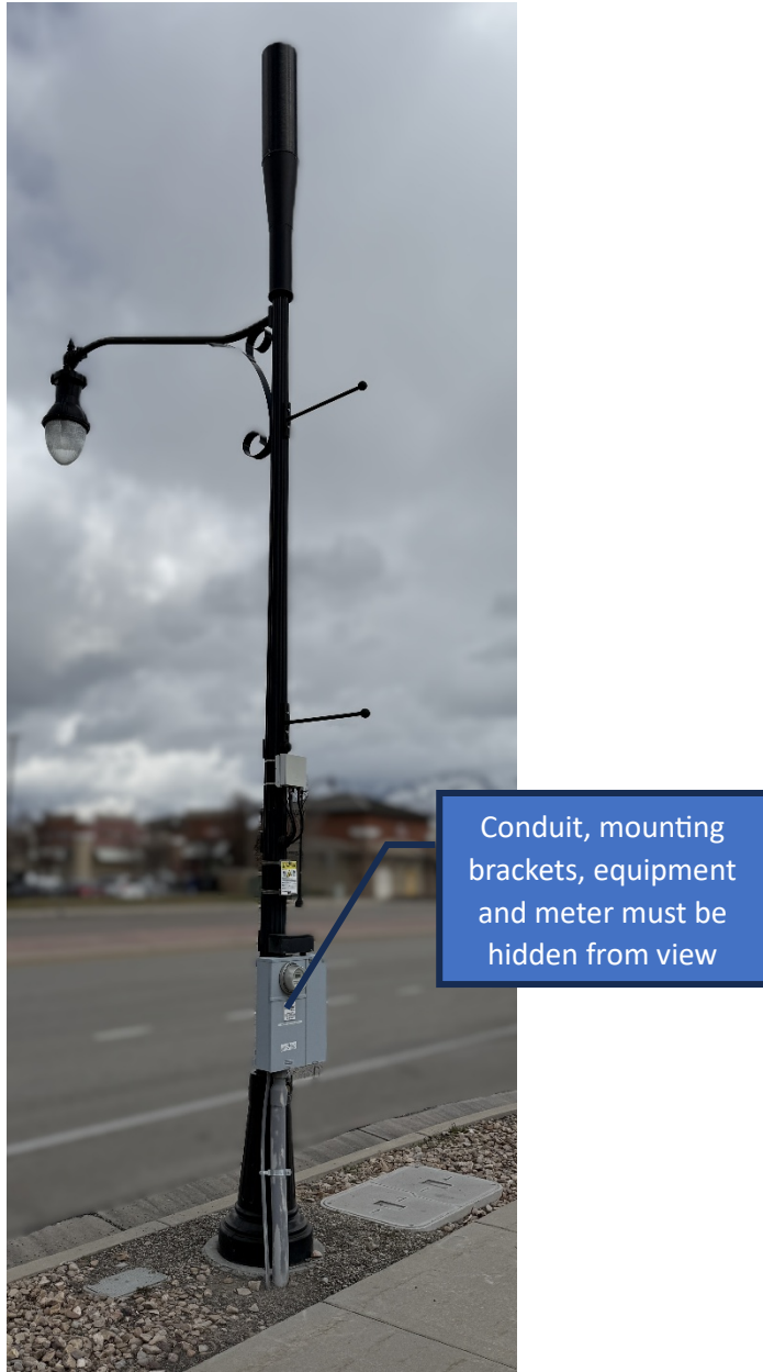
Figure 3: Unacceptable Type 2 Installation
