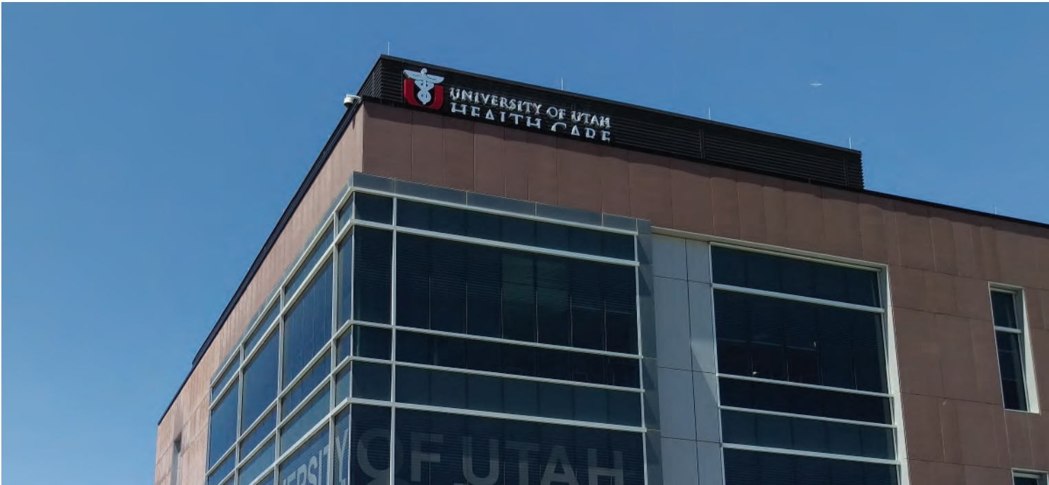
Parapet Building Signs
